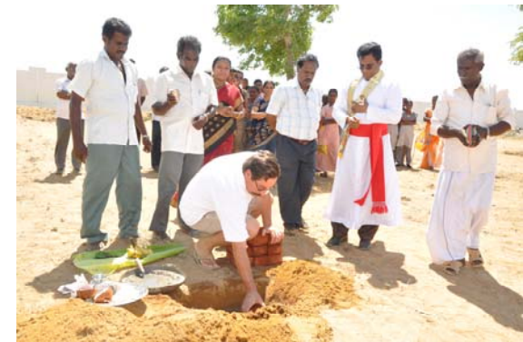
First bricks are laid.
